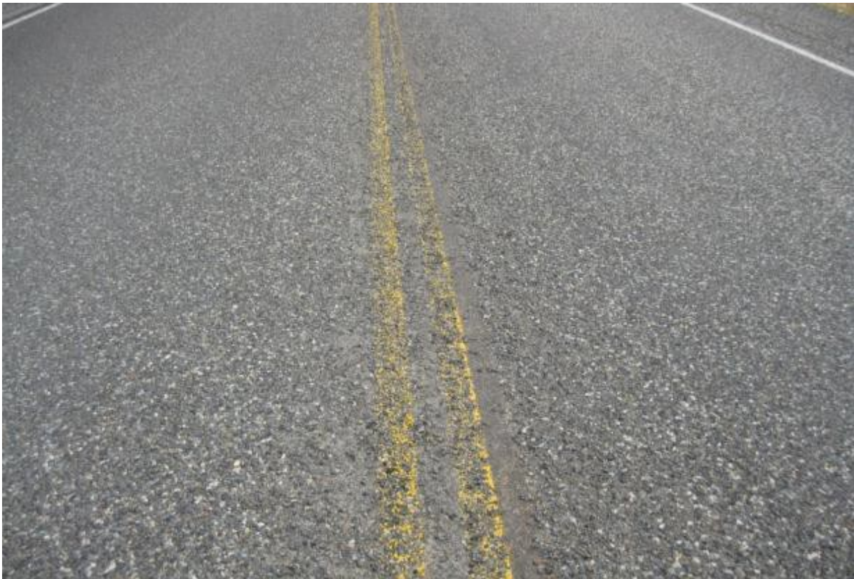
Longitudinal Joint: Acceptable chip loss
