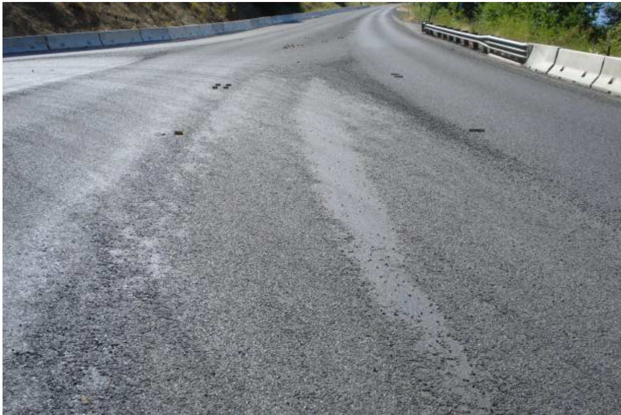
Traffic: Chip loss from turning movements (CODS)
