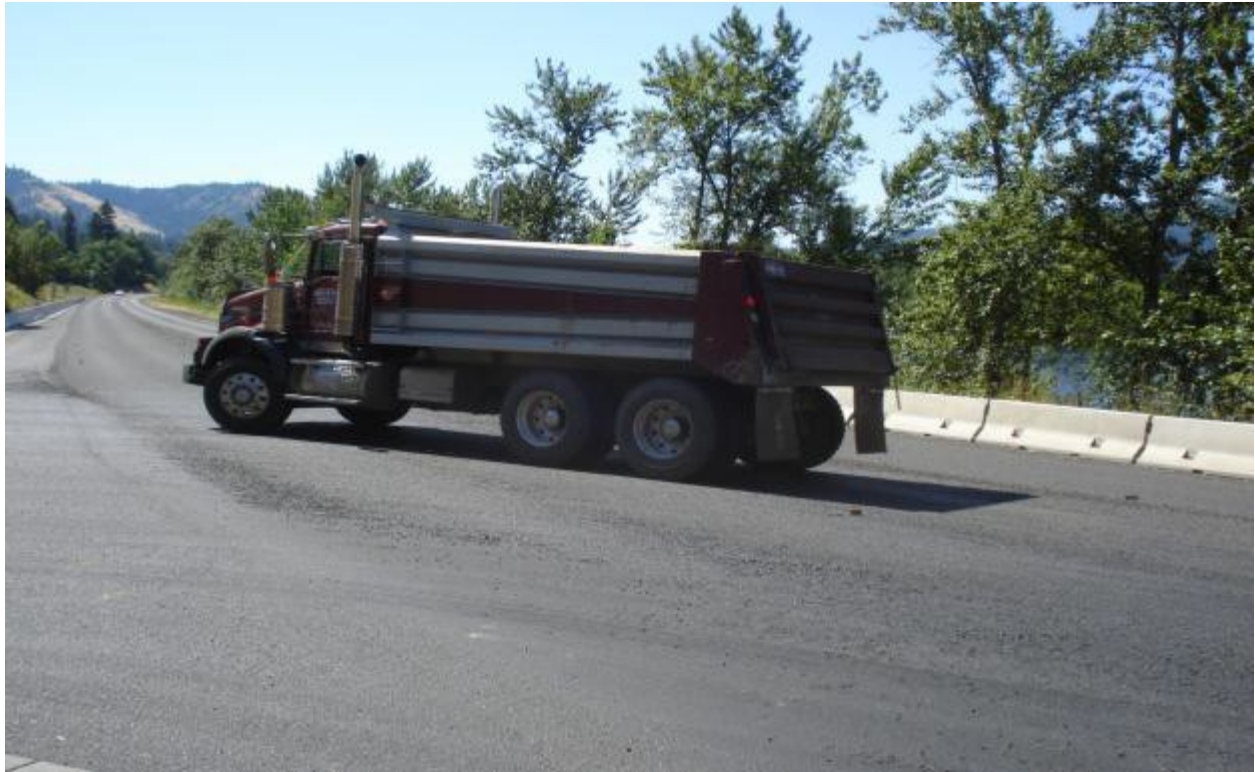
Traffic: Chip loss from turning movements (CODS)
