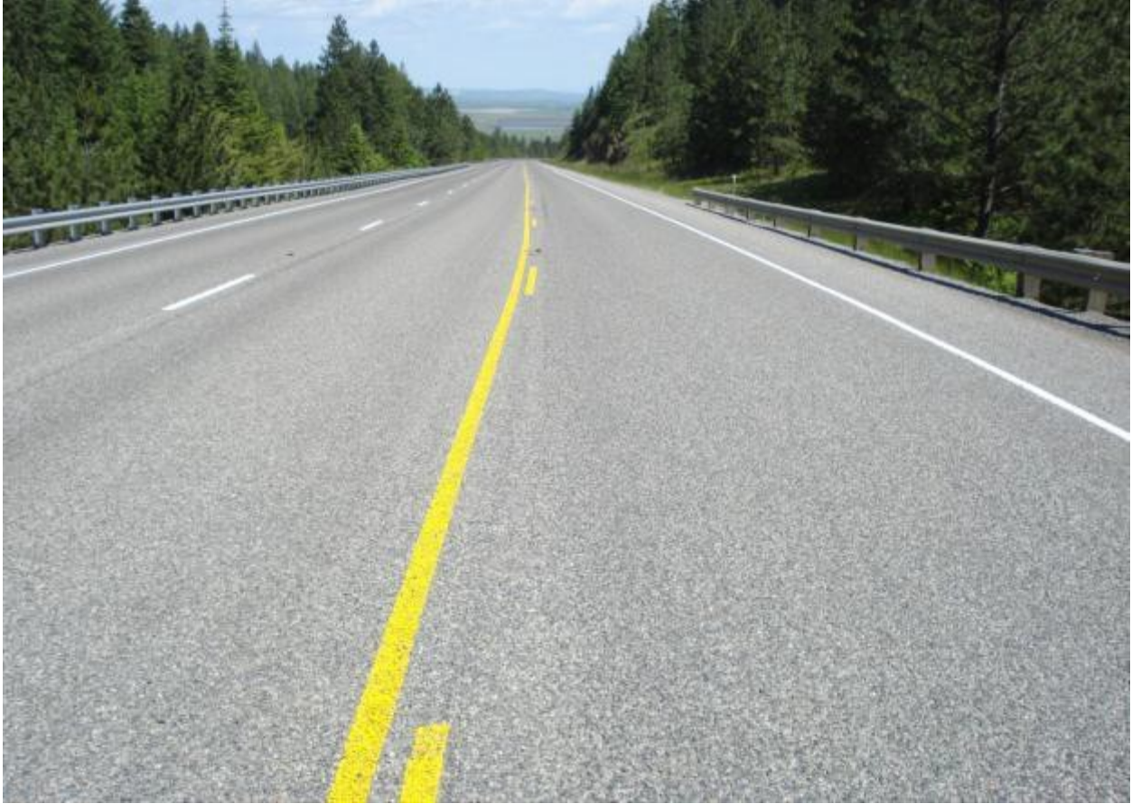
US-95, Milepost 232. Looking north from Whitebird Hill A desirable Sealcoat
