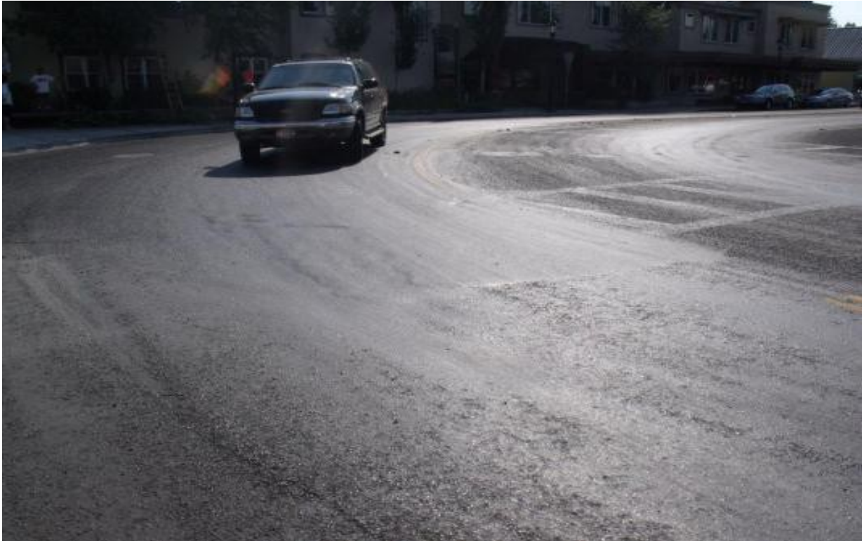
Traffic: chip loss from turning movements (CODs)
