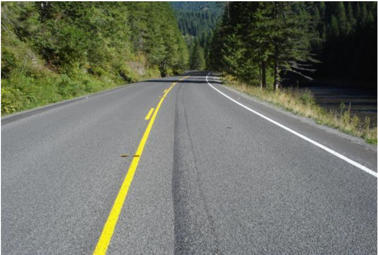
Plugged nozzle: Acceptable repair
