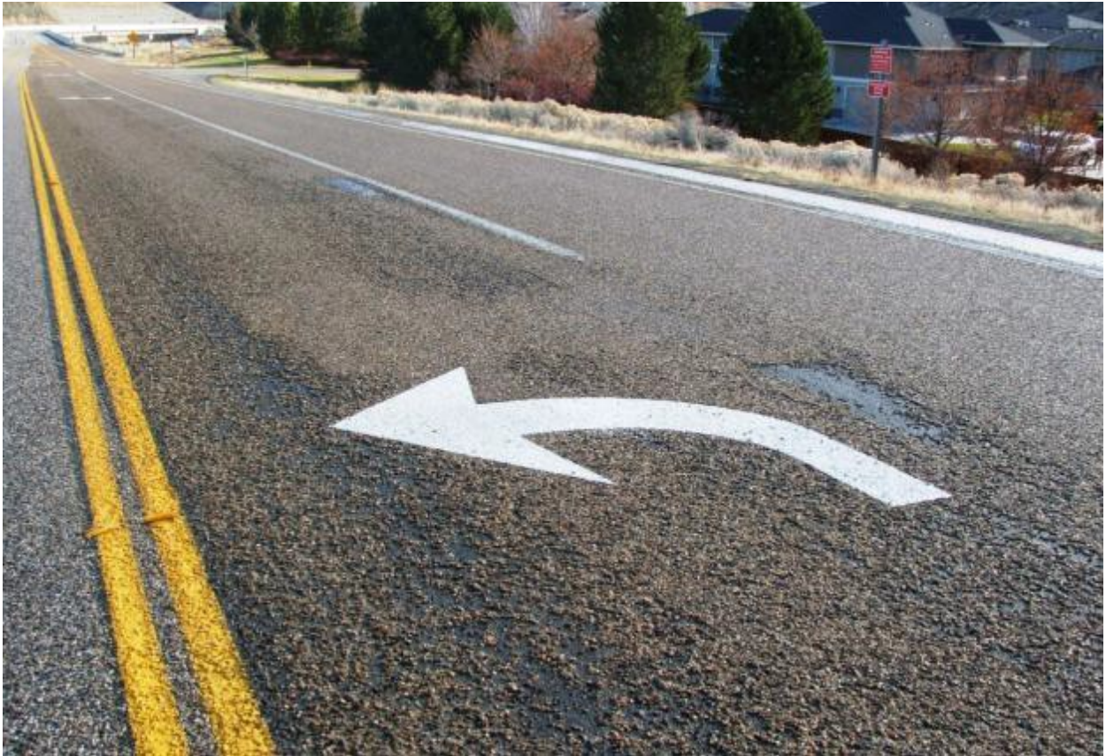
Design: Sealcoating on newly paved asphalt pavement: Unacceptable chip loss (CODs)
