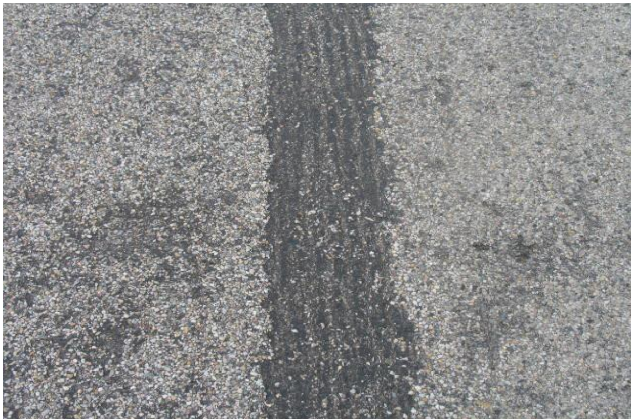
Traffic: Tire chain damage (NCODs)
