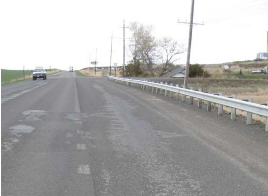
Snowplow: CODs Exacerbated by Snowplows - Unacceptable
