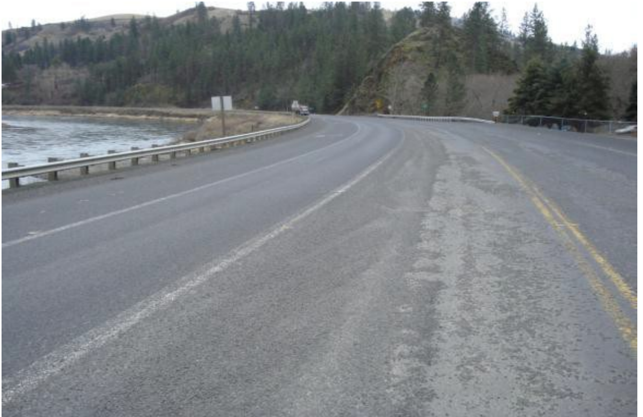
Design: Sealcoating on newly paved asphalt pavement: Unacceptable chip loss (CODs)
