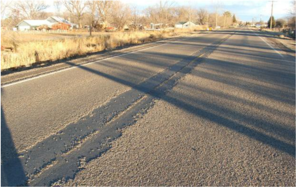
Longitudinal Joint: Unacceptable chip loss (CODs)
