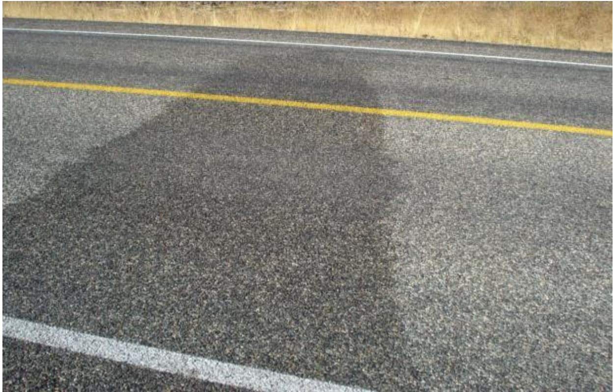
Traffic: Tire chain damage (NCODs)
