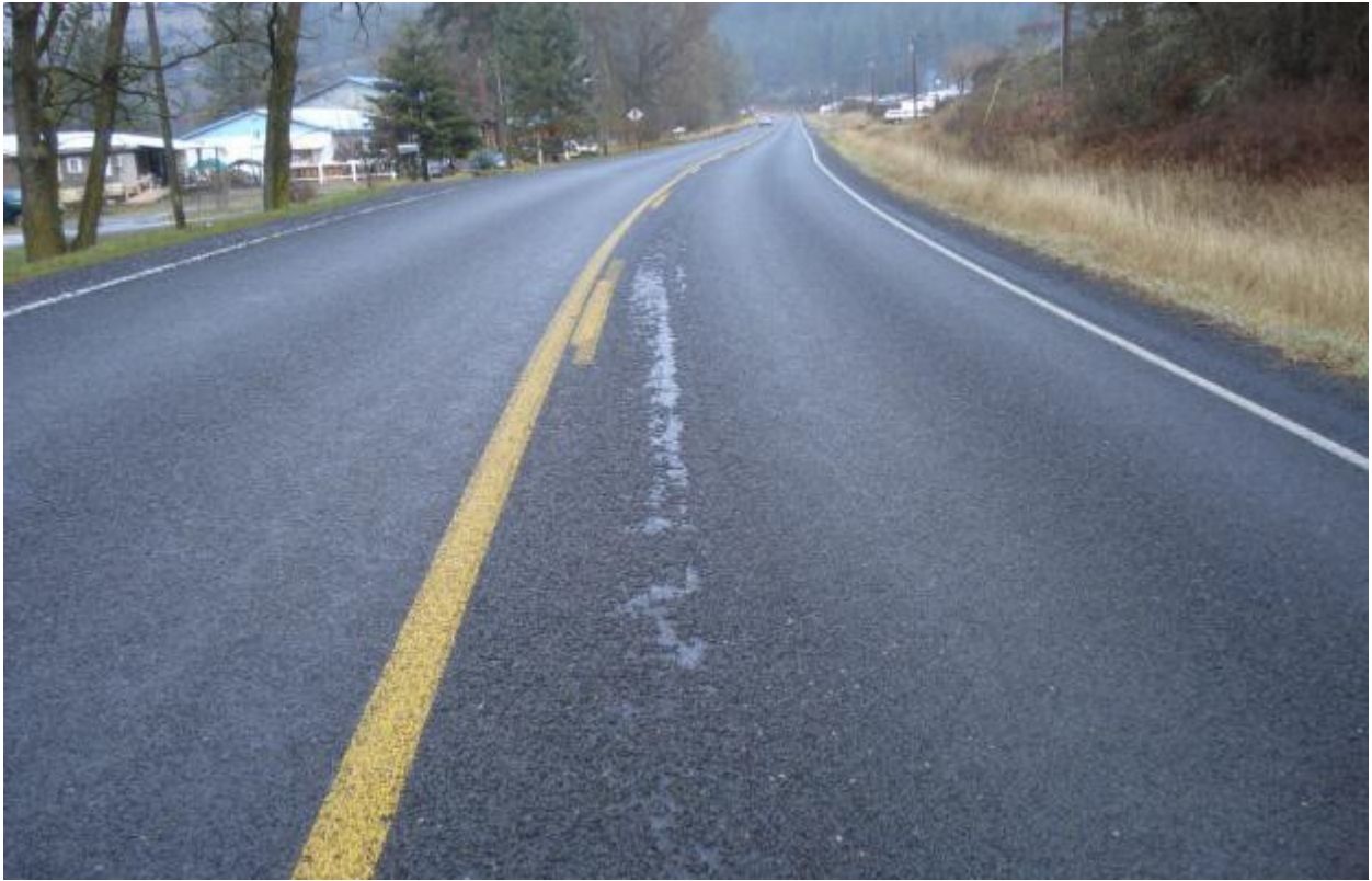
Plugged nozzle: Acceptable repair
