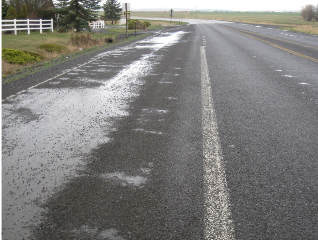
Snowplow: CODs Exacerbated by Snowplows - Unacceptable
