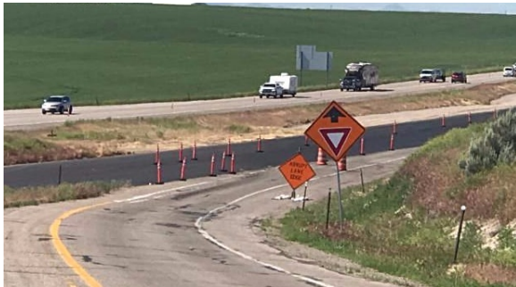
Exit 108, Bonneville County
