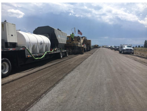
Paving equipment on I-15 between Arimo and McCammon
