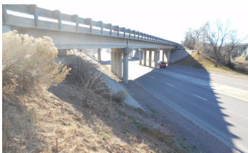
S. 5th Avenue Bridge
