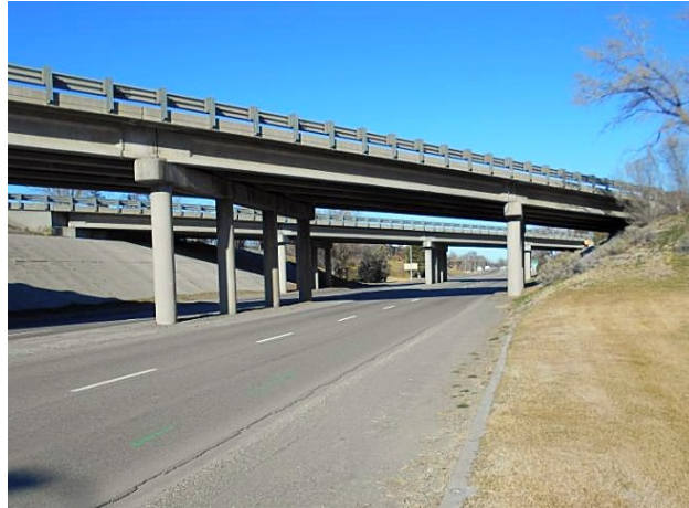
East side of S. 5th Avenue where the sidewalk is planned
