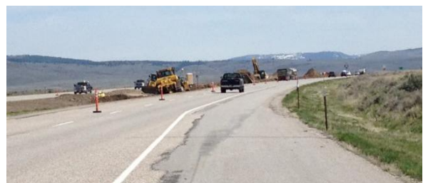
Crossovers will allow all traffic to use southbound I-15 while the northbound lanes are resurfaced.
