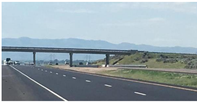
ITD replaced 3.6 miles of pavement south of Blackfoot.
