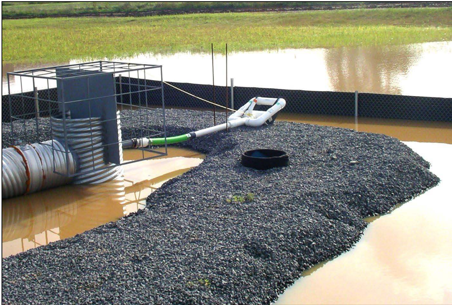
Figure 3. Photo showing example of a riser, trash rack, anti-vortex device, skimmer and landing pad.
