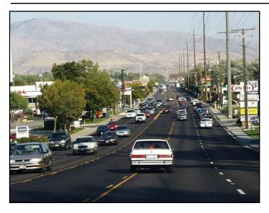
**2.1.3 Two Way Left Turn Lanes (TWLTL)** TWLTL have been shown to be effective in reducing left turn and rear end accident rates in many applications. In urban and suburban applications, the reduction may be as much as 35%. The accident reduction in rural applications is not as dramatic, but if properly used at higher crash locations the TWLTL can have a large effect.
