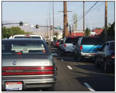
The overall lane width of a roadway influences the safety and comfort of the driver as well as the overall performance of a roadway. The 12 ft. lane provides desirable clearances between larger commercial vehicles traveling in opposite directions.
