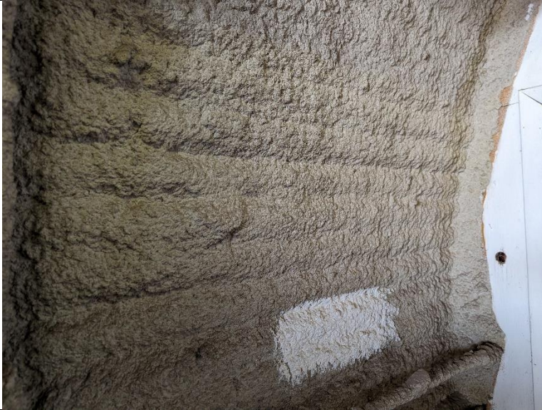
17) Insulation/Fireproofing – Workshop – Not ACM
