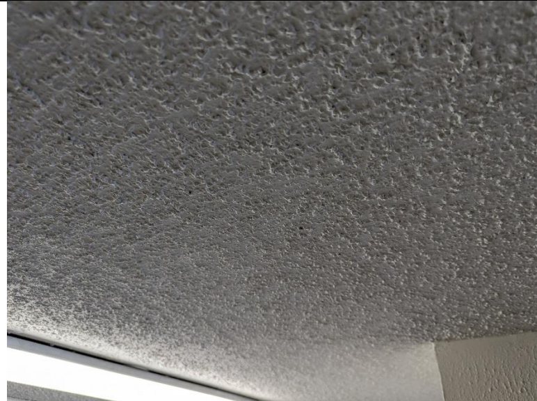
20) Popcorn Ceiling Texture – Hallway
