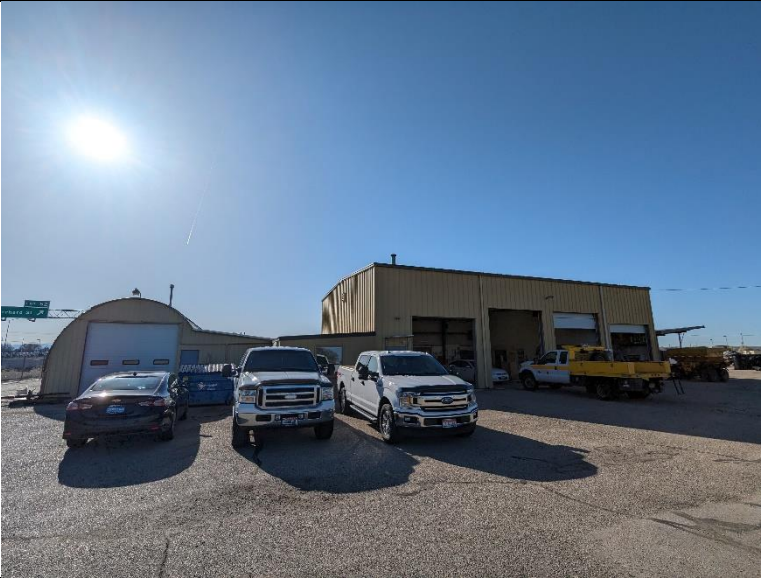
1) ITD Shed – 2666 S Eagleson Pictured from the West
