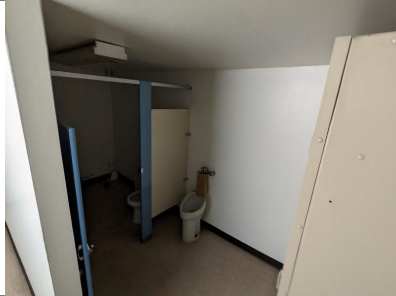
10) Breakroom Area Bathroom
