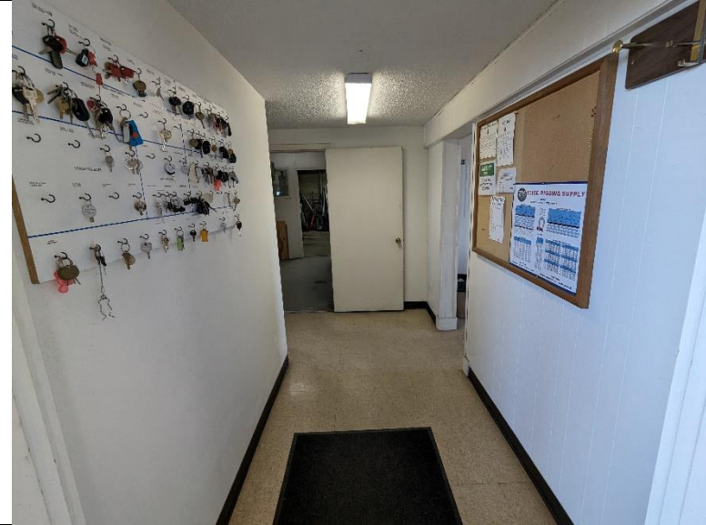
6) Hallway – Vinyl Tile(5% Chrysotile) found underneath visible tile is ACM
