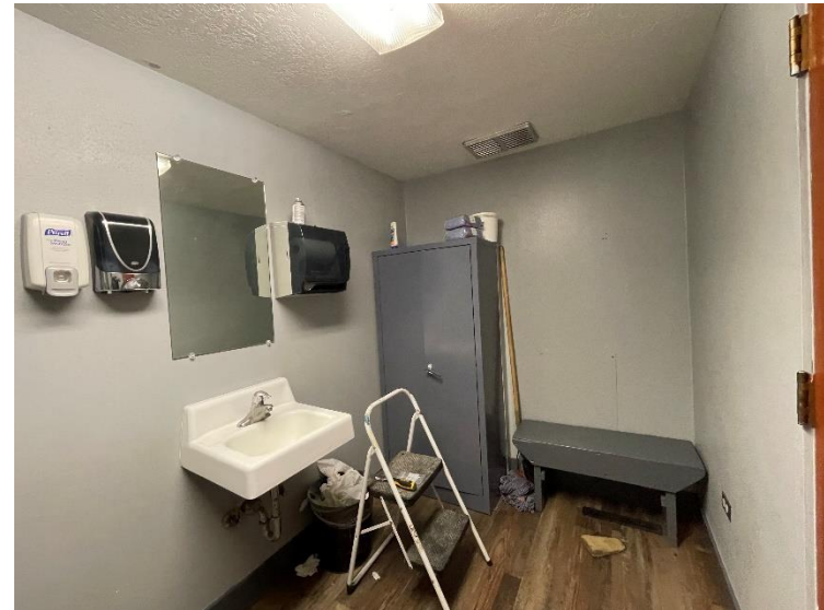
4) Bathroom-Sample 3-7 was taken from here-No ACM
