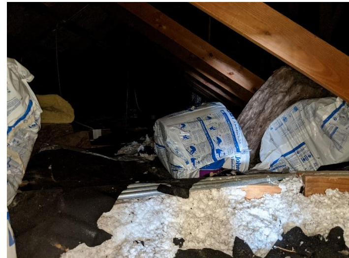
4) Attic – Loose Fill Insulation and Tar Paper
