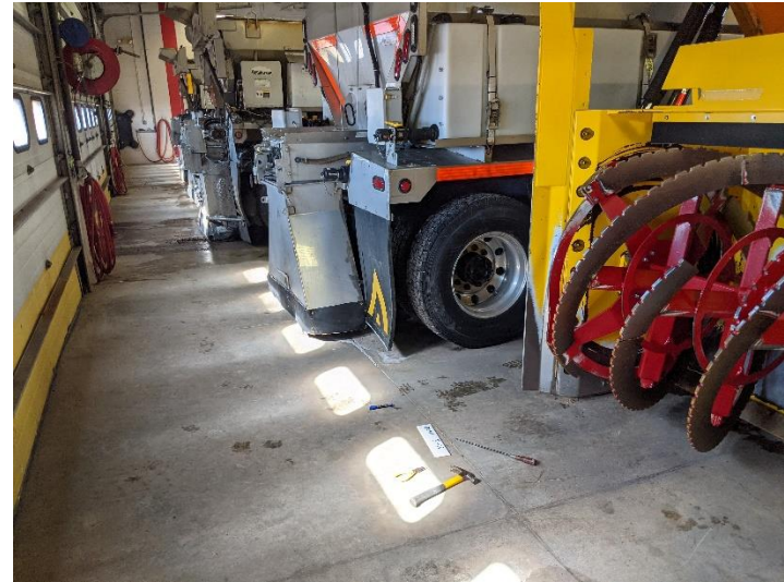
2) Garage Bay 2 – Concrete Foundation
