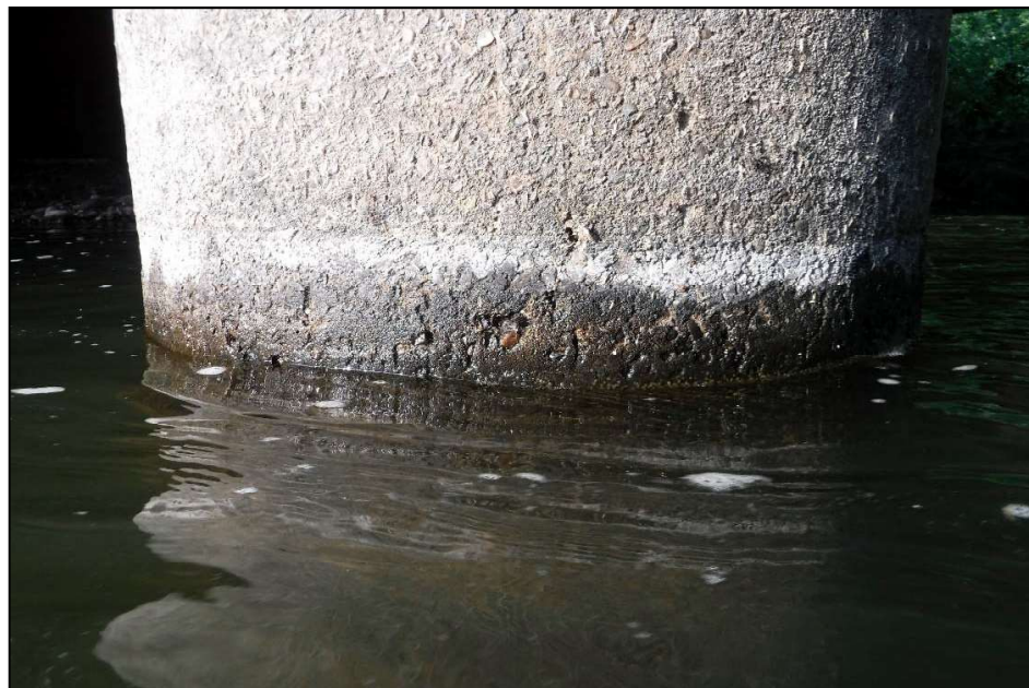
Photograph 3: Typical Condition of Concrete at the Waterline.
