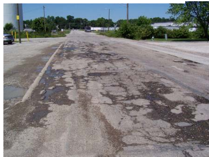
Figure 25: Pavement at 0.0 Crack Rating
