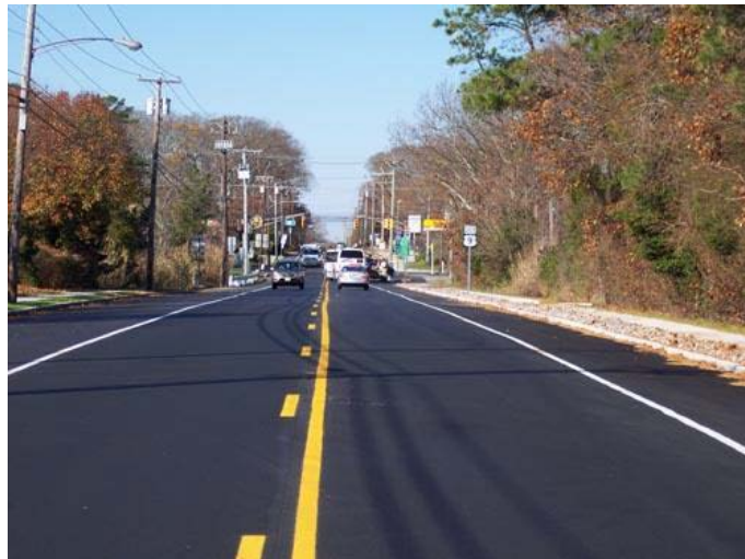
Figure 24: Pavement at 5.0 Crack Rating
