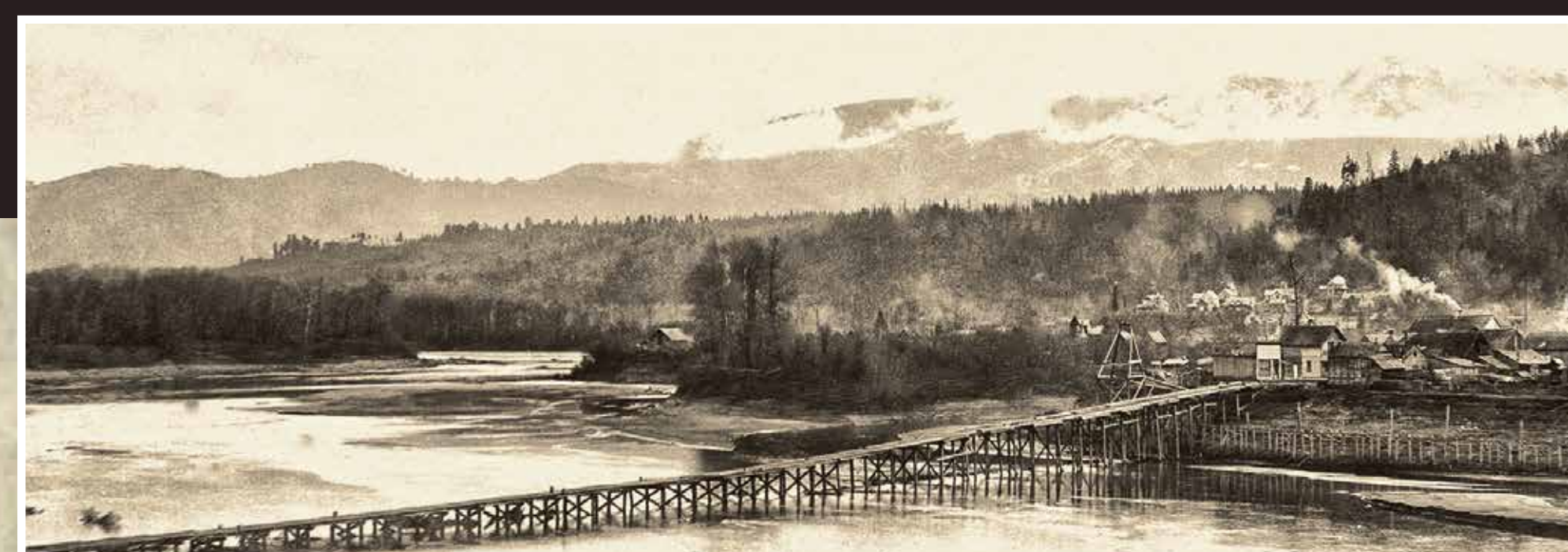
The low water bridge built in 1905 was impassible during high water in spring and early summer. When the center of the bridge was under water, the ferry filled the gap. Dynamite was used to break up logjams and the bridge had to be repaired every year after floodwaters receded.
