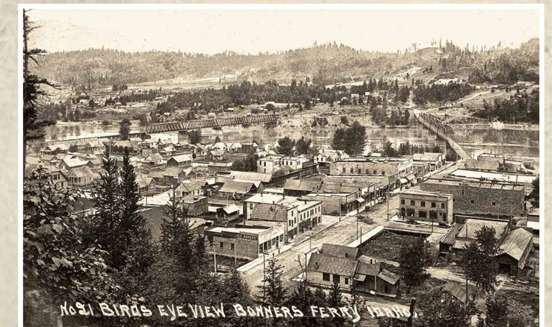
This photo of Bonners Ferry gives a "birds eye view" showing both the Spokane International Railroad bridge (left) and the 1910 bridge (right).
