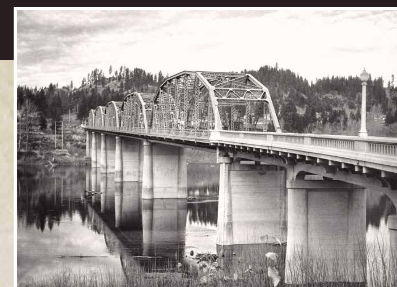
When the five-span steel girder and concrete bridge was completed in 1933, it was Idaho's longest bridge. One hundred-fifty men worked five-hour shifts to complete the $200,000 Public Works project in a record-setting four and a half months! This new bridge included the pedestrian walkway its predecessor lacked. You are standing on the approach of the old 1933 bridge.
