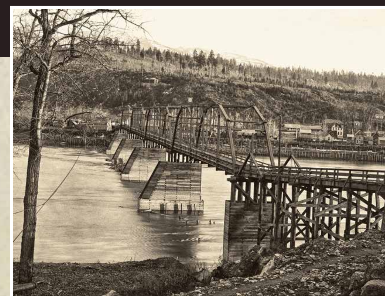
The 1910 "high bridge" was constructed of wood and steel. Unable to raise $1,100 for a wooden sidewalk on the bridge, citizens were told, "You will have to cross the bridge in the middle or walk along the side." A woman was once knocked off the bridge by a careless driver. Signs on the bridge limited speed to no faster than a walk for horses and 10 miles per hour for motor vehicles. The weight limit was six tons.
