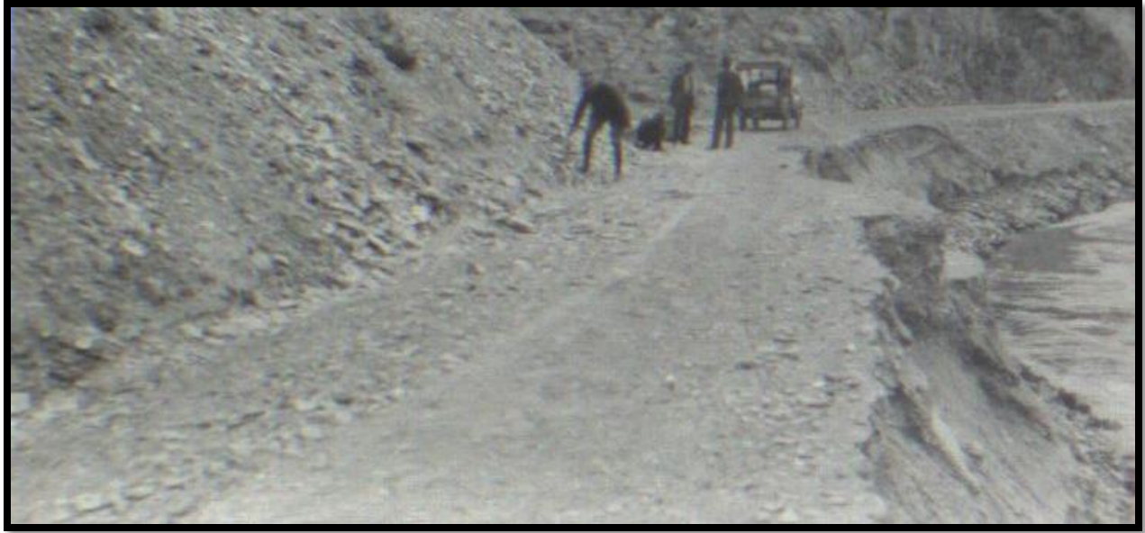
Figure 20 Rock slide and shoulder slough along the Little Salmon River 142
