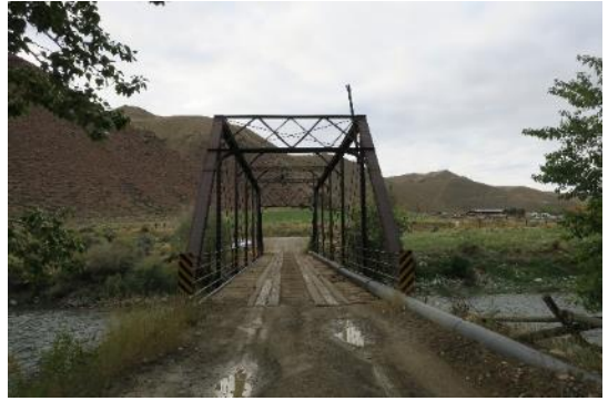
Salmon River Pratt Truss Bridge at Bayhorse Creek (37-005784/ITD Key# 31660)
