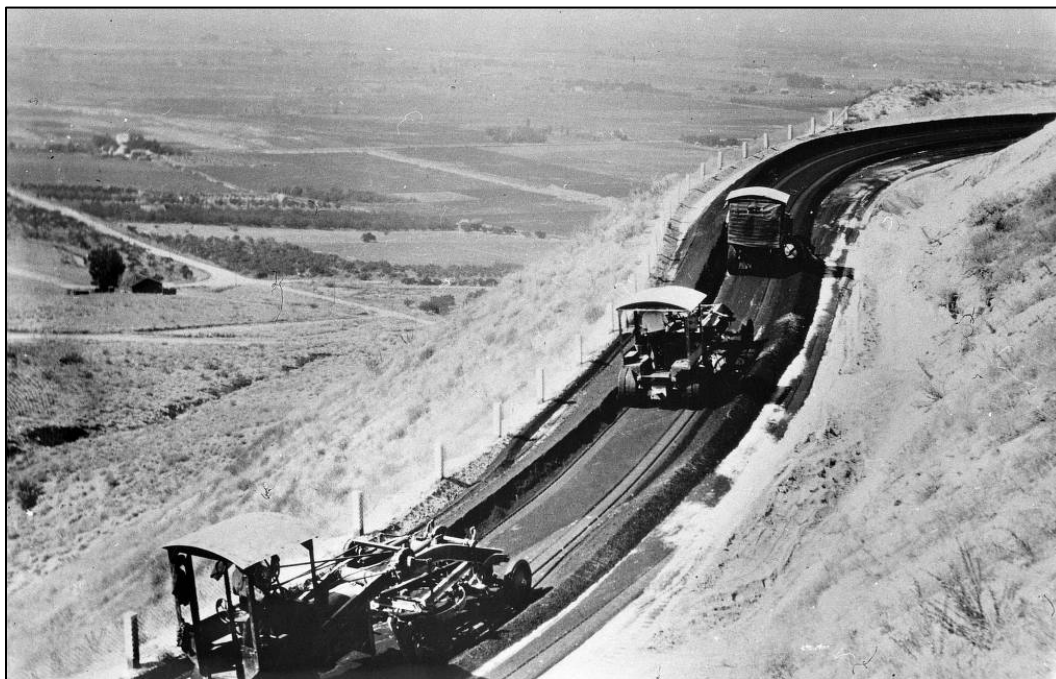
Figure 39. Mixing oil into surfacing material, Freezeout Hill, Gem County, 1930.. 256
