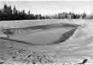
Uned sediment basins are used to collect runoff from distulbed areas on construction allies and allow heavier solids to settle out.
