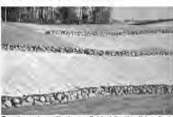
Tenscing can be used to slow runoff. Lined diversion dilches direct flow away from exposed areas toward stable portions of the site.
