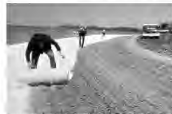
Exposed soils are very vulnerable to erosion. Mulch or other ground cover protects surfaces from wind and storm water erosion, as well as slowing vegetative growth.
