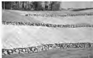
Trenching can be used to slow runoff. Lined diversion ditches direct flow away from exposed areas toward stable portions of the site.
