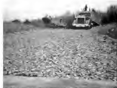
Stabilized construction entrances allow dirt to be removed from the tires as trucks leave construction sites.
