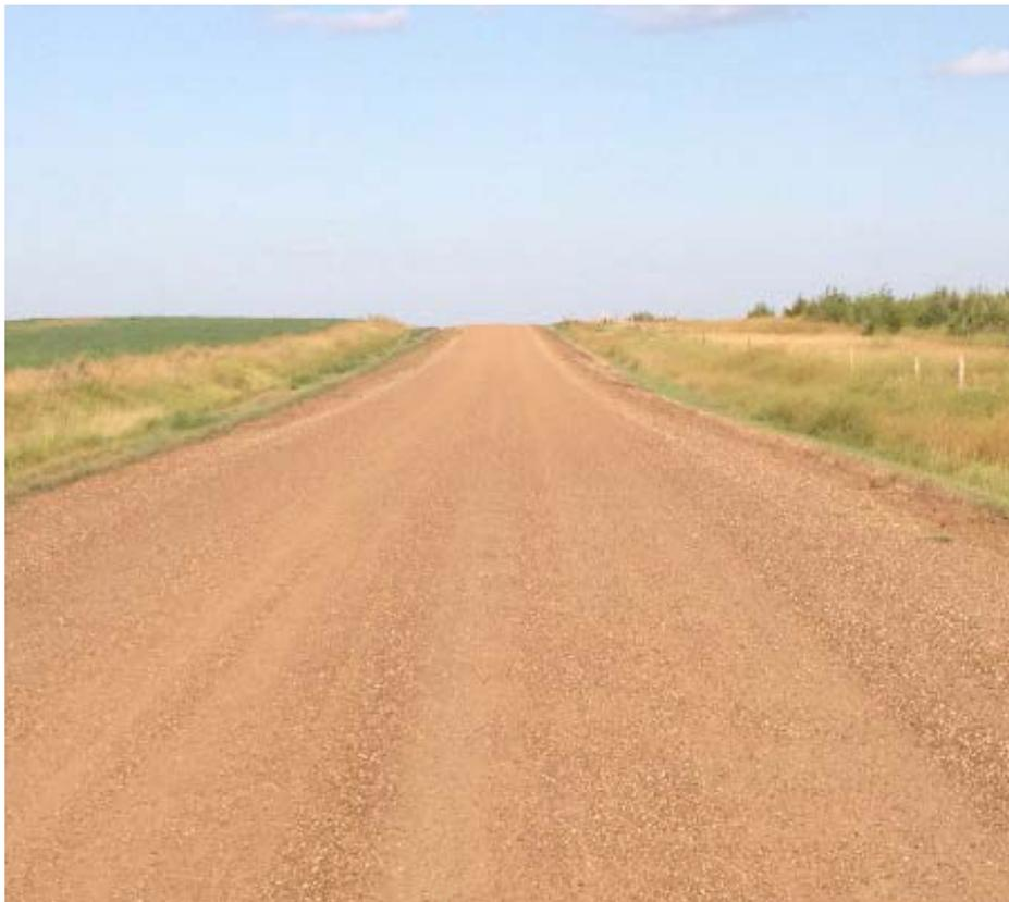
Figure 8: Gravel road with adequate crown.
