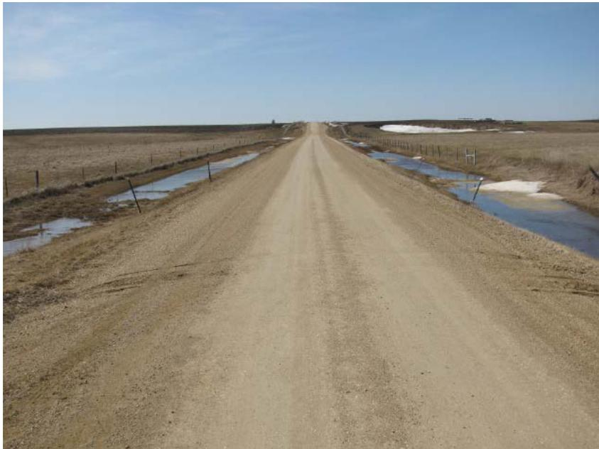
Figure 10: Gravel road with excessive crown.
