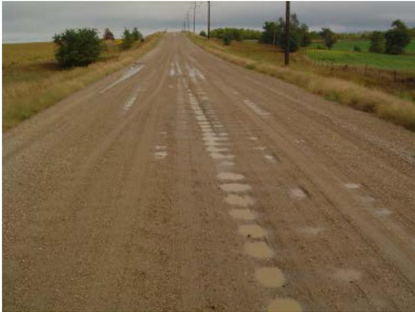
Figure 9: Gravel road with inadequate crown.
