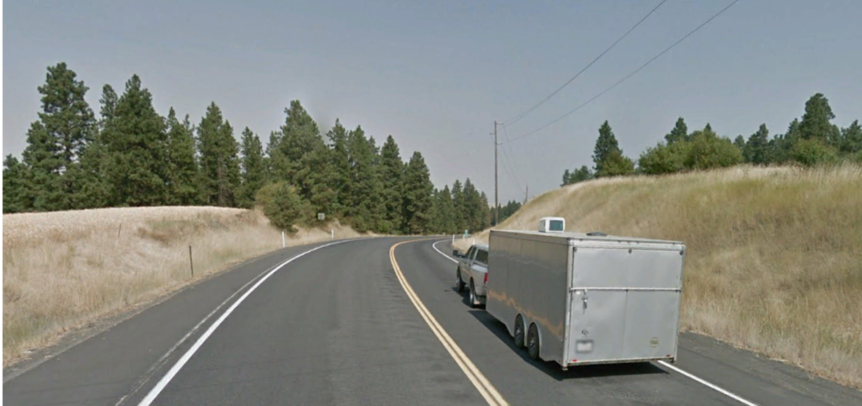
Photo: Existing Inadequate Passing Sight Distance at the Crest of Crooks Hill and Potential Risk of a Dangerous Passing Maneuver
