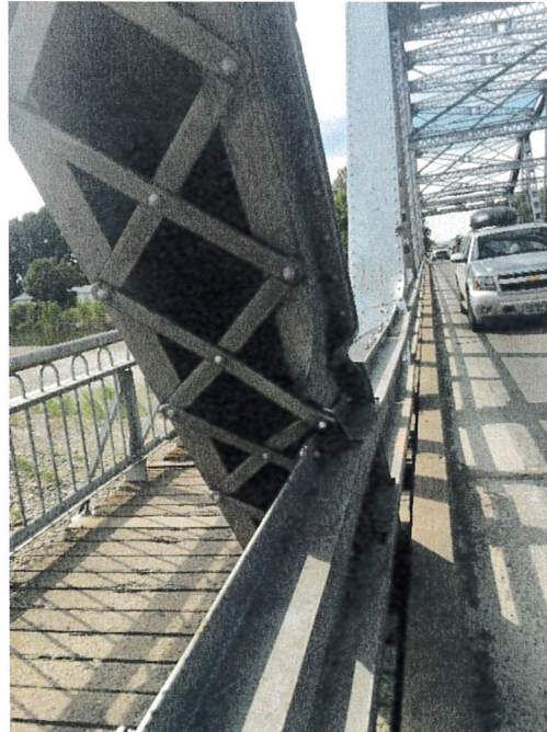
Figure 3. Example Girder Damage
