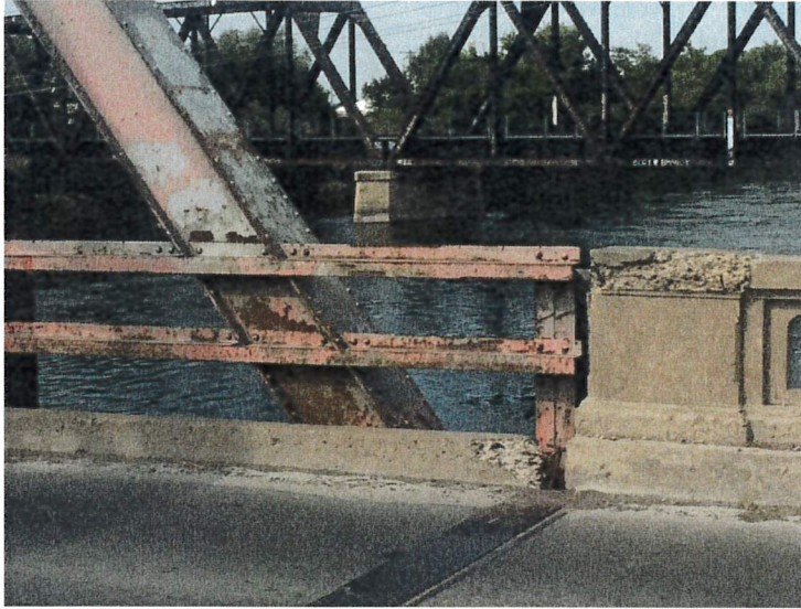
Figure 4. Deteriorated Concrete and Paint
