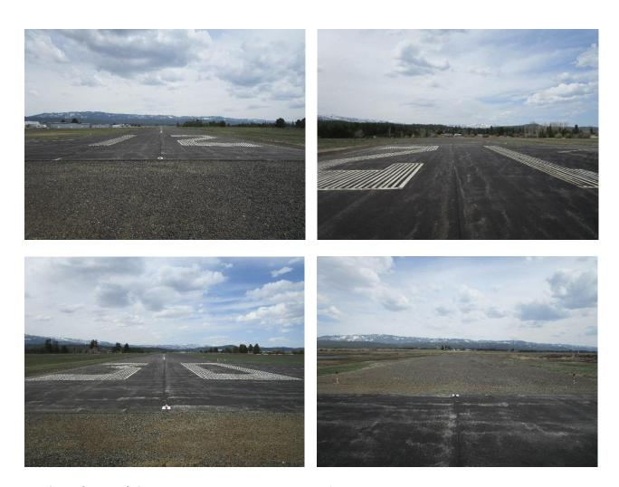
Taxiway/Ramp/Tiedowns: The taxiway at this facility was in good condition and displayed good markings. Vegetation was well kept and under control. The parking apron/tie down area was in poor condition and had major cracks that have become elongated depressions with grass growing out of and through them. Of the 25 available parking spots, 5 had tie-down chains present. I am excited to see your new ramp later this summer after it gets rehabbed.
