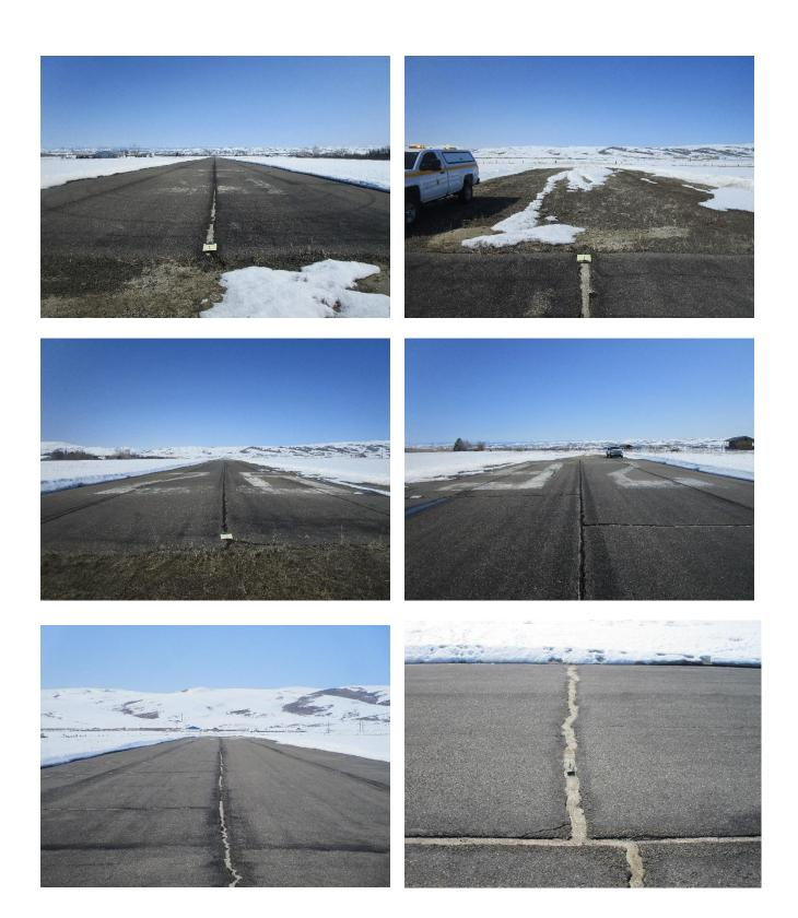
**Taxiway/Ramp Tie-Down:** There is no taxiway at this facility. Tie down area had mostly good surface and fair paint markings. There are a few areas where the pavement is coming apart and small chunks of asphalt are becoming FOD (foreign object damage) for the area (see pics). Vegetation around the runway and the tie-down area was still under snow cover, but it appears to be well managed and under control.
