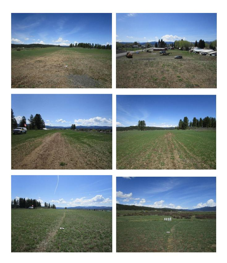
**Boundary Markers (BMs):** The painted rock boundary markers were in good shape and had good paint coverage (75-80% paint left). They were clear, free of vegetation and visible from the air. Not this year but in a couple of years, some new paint on the boundary markers and the segmented circle around the windsock would help and sharpen things up.
