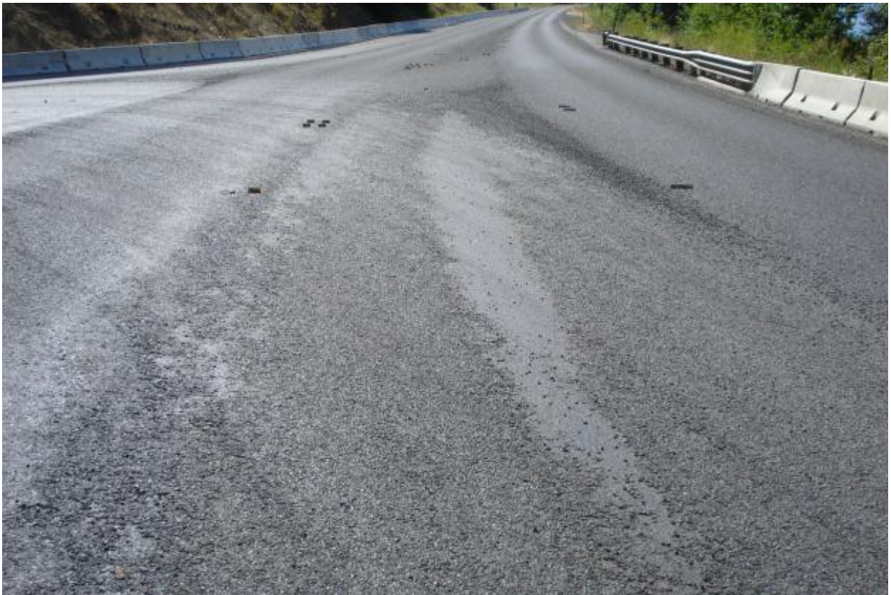
Traffic: Chip loss from turning movements (CODs)
