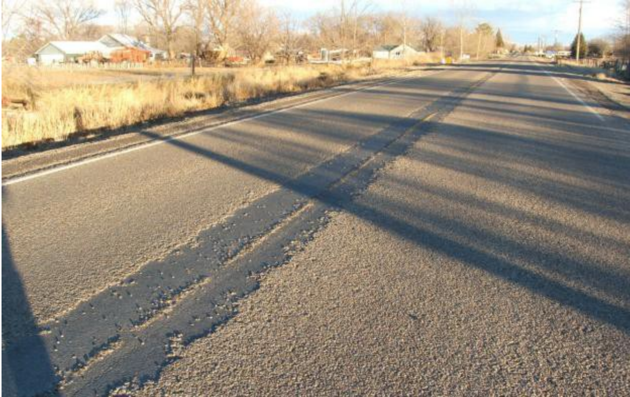
Longitudinal Joint: Unacceptable chip loss (CODs)
