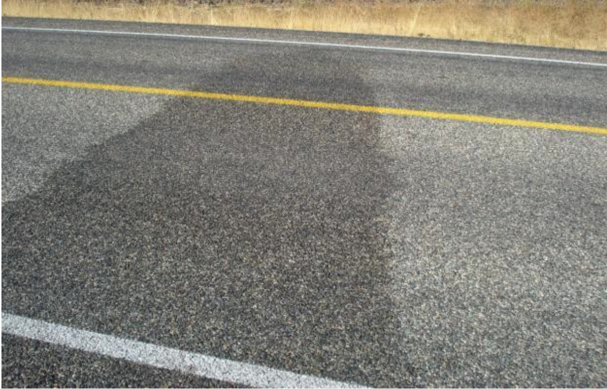
Traffic: Tire chain damage (NCODs)
