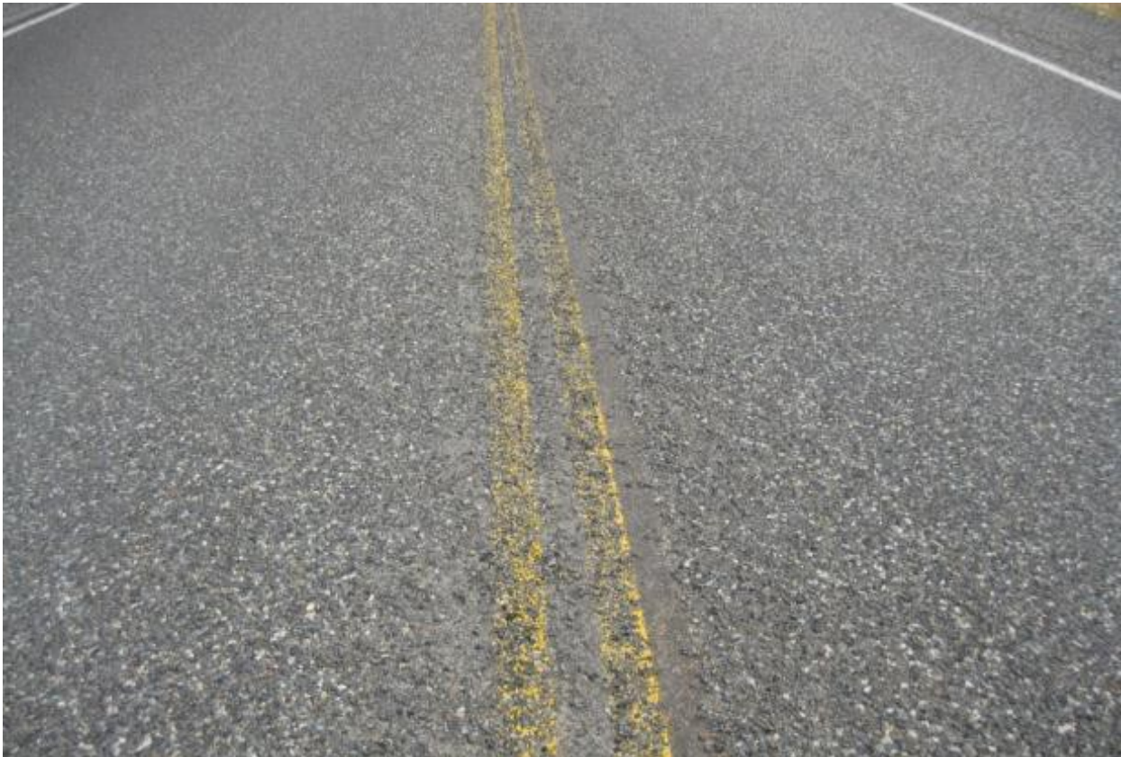
Longitudinal Joint: Acceptable chip loss
