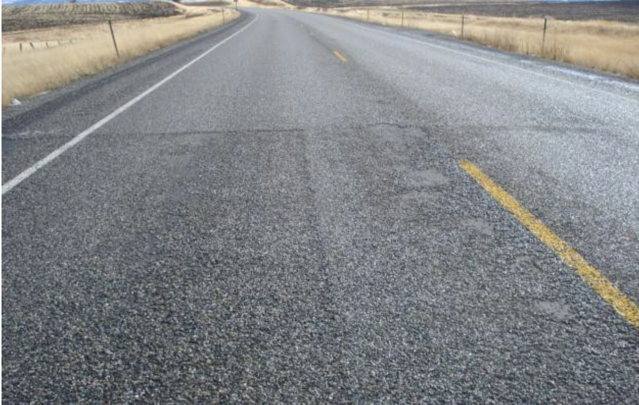
Transverse Joint: Acceptable chip loss
