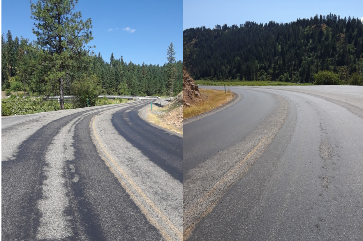
Catastrophic Chip Seal Loss
