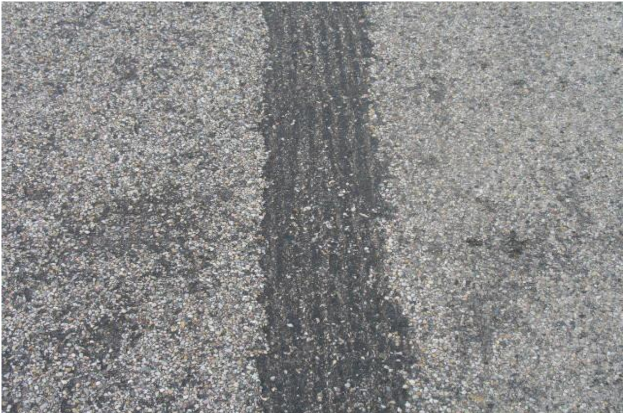
Traffic: Tire chain damage (NCODs)
