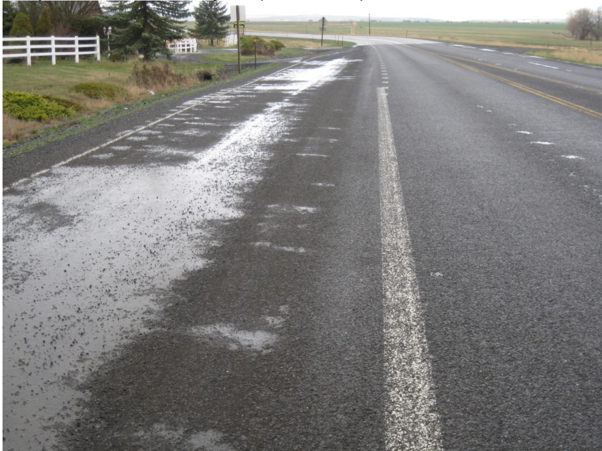
Snowplow: CODs Exacerbated by Snowplows – Unacceptable
