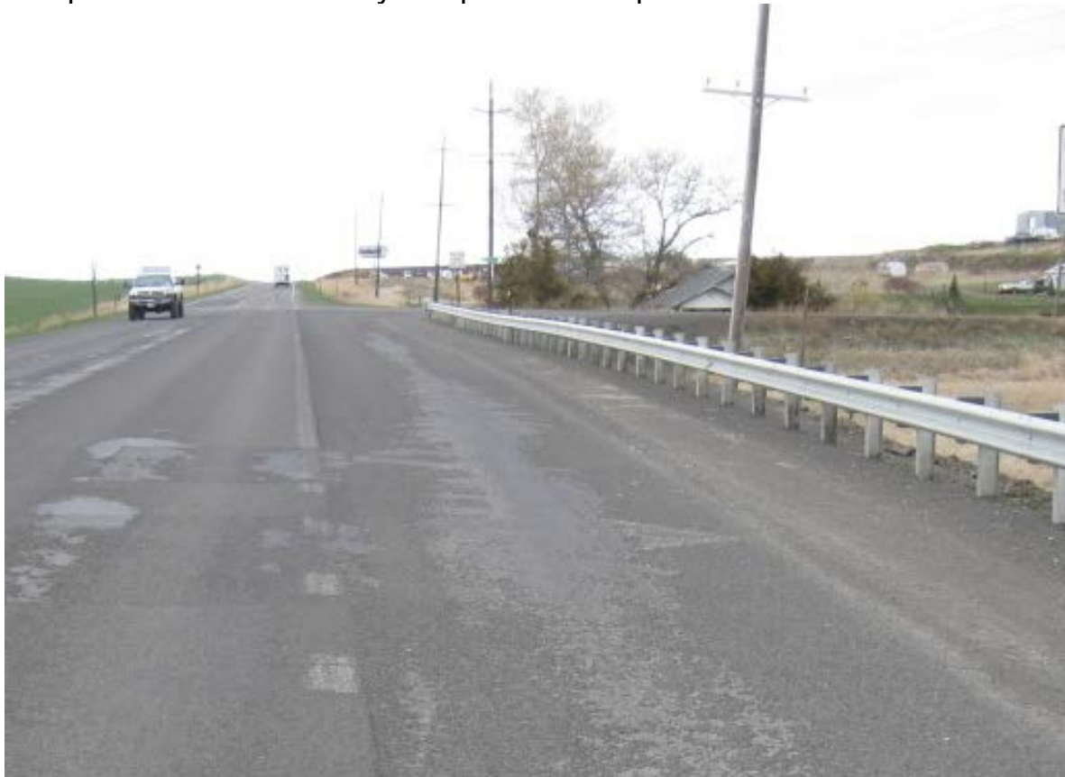
Snowplow: CODs Exacerbated by Snowplows – Unacceptable
