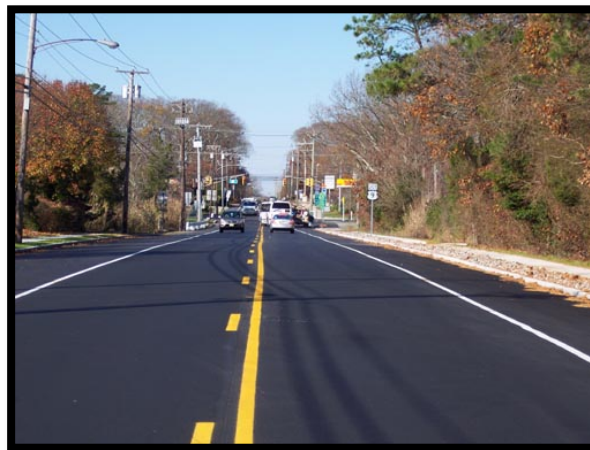
FIGURE 22: EXAMPLE OF 5.0 CRACK RATING
