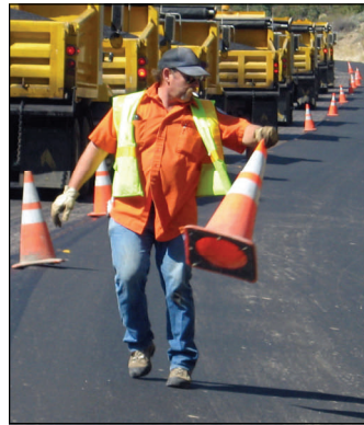
Gary Cvechich tossing cones during Idaho 75 paving on Sept. 17
