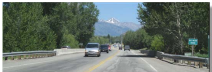
Existing two-lane Big Wood River Bridge
