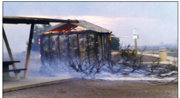
Below: The pump house at the Jerome Rest Area on Interstate 84 went up in smoke along with several bushes and trees during a wild fire on July 6, as captured here by Scott Malone.
