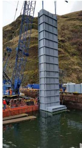
Installing a supplemental water intake chimney for the fish ladder at Lower Granite Dam.
