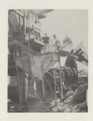
Figure 3 - Asbestos Mixing at Hotmix Plant
