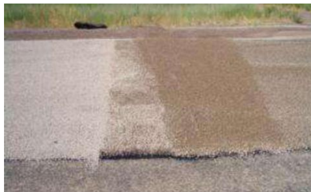
Figure 7. A Segment Where Chip Seal was Applied Twice
