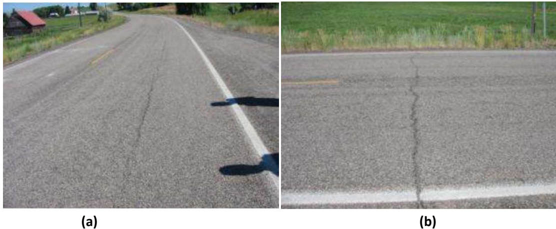
Figure 6. (a) Longitudinal and (b) Transverse Cracks Observed Before Chip Seal Application
