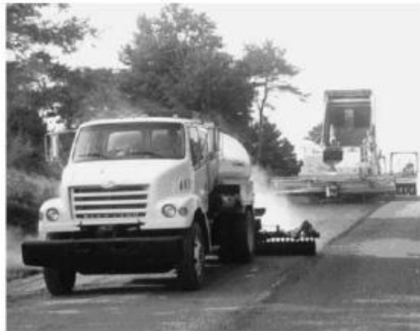
Figure 4. Asphalt Binder Sprayer Followed by Aggregate Spreader Truck (2)
