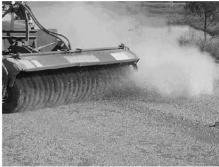
Figure 2. Rotary Brooming Process (2)
