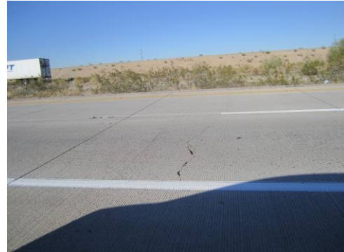
Transverse Fatigue Cracks JPCP
