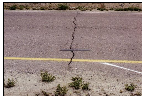
Transverse Cracks HMA
