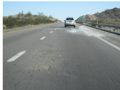
Alligator Fatigue Cracks HMA
