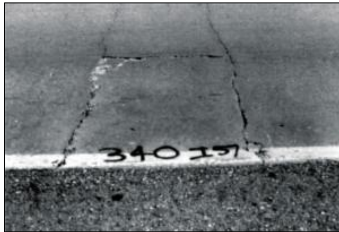
Figure 5 Edge Punch-out in CRCP
