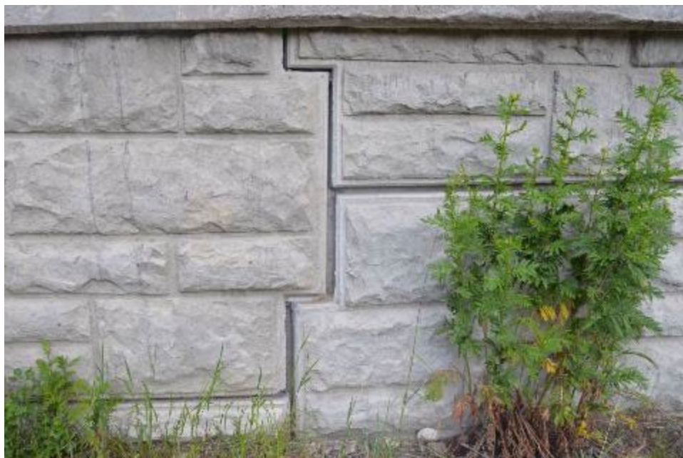
Figure 9. Rotated Panel at L = 30 feet
