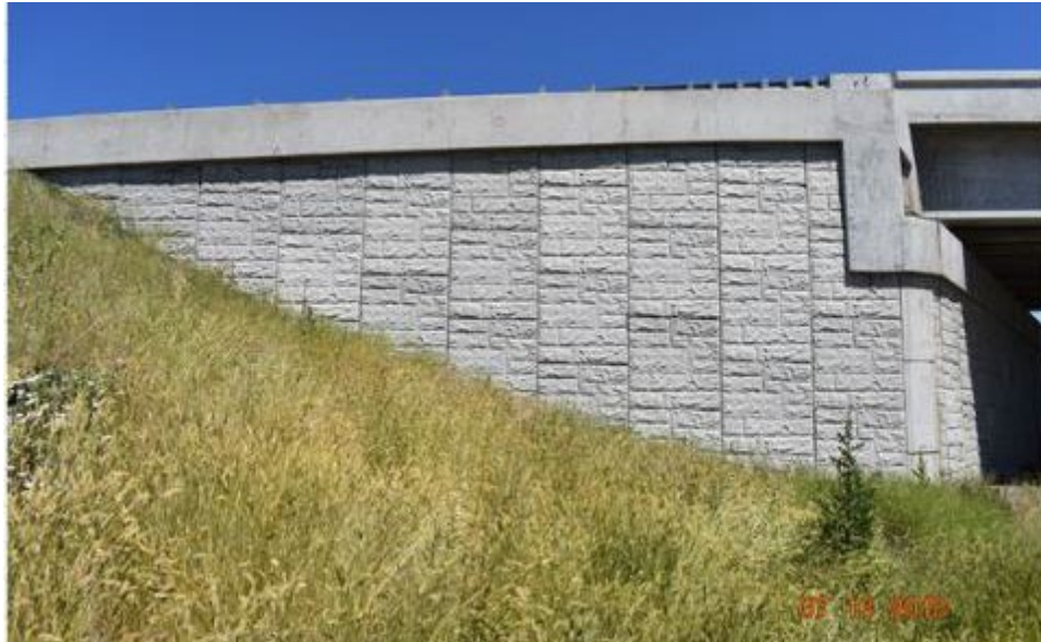
Figure 88. South MSE Wall, West Abutment of SH-33 Exit at US-20
