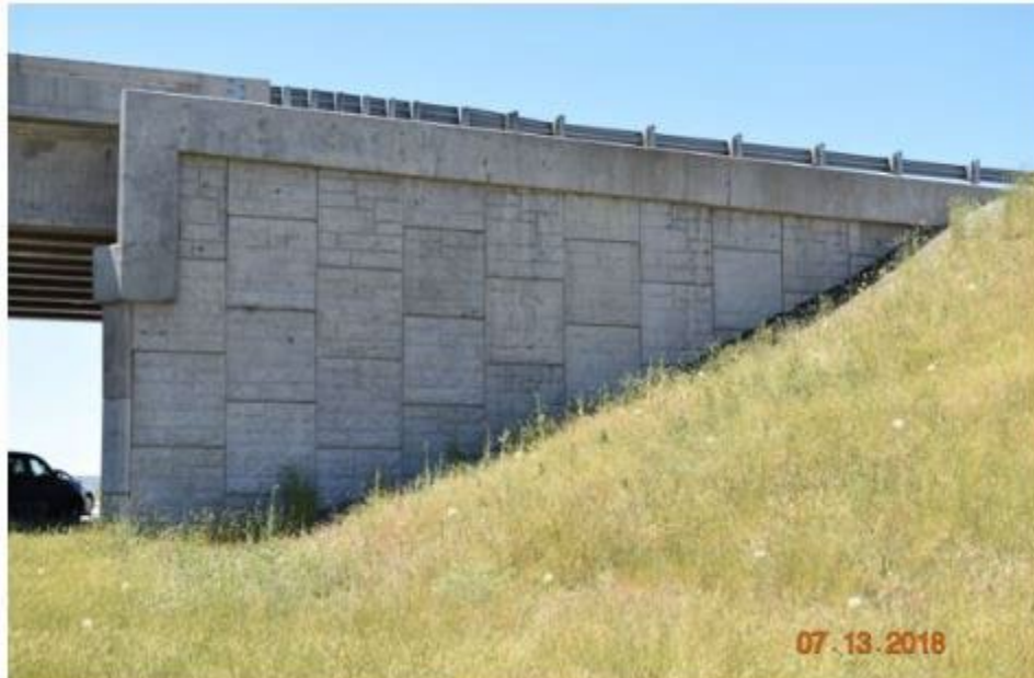
Figure 90. North MSE Wall, West Abutment of SH-33 Exit at US-20
