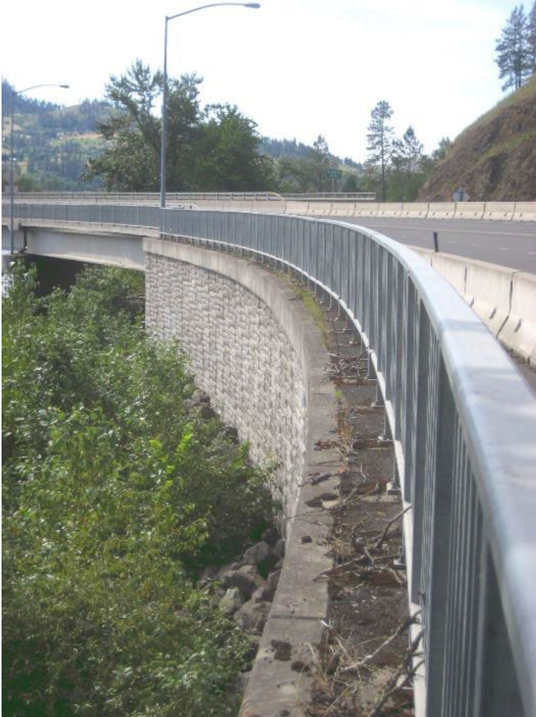
Figure 20. Closer View of Eastern MSE Wall of Kamiah Bridge from the Deck
