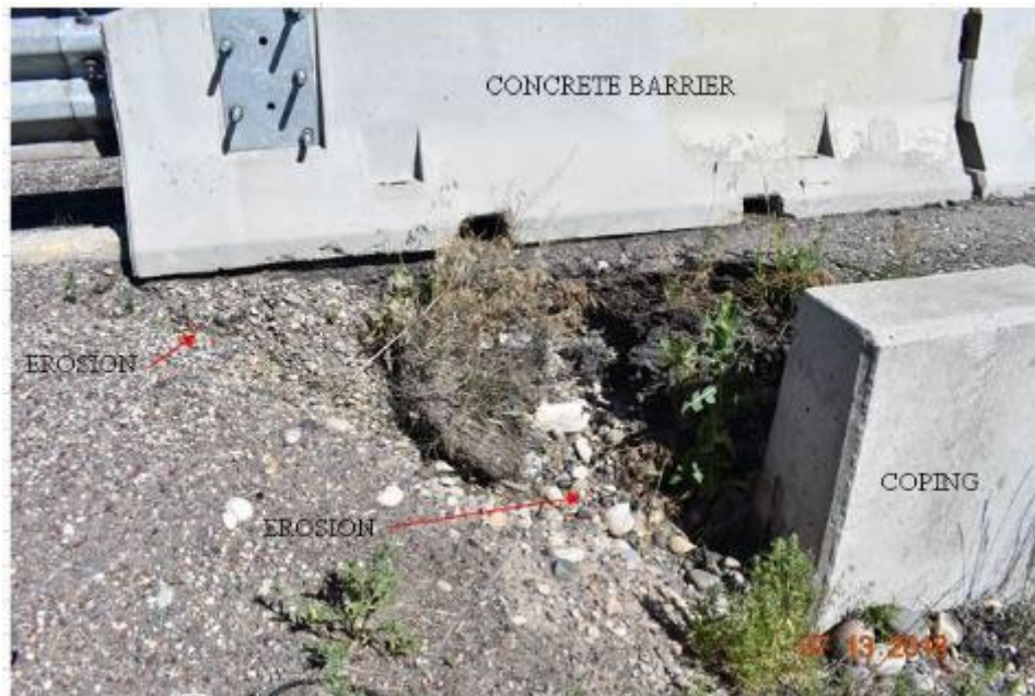
Figure 78. Erosion Channel at Edge of South Wall, West Abutment, US-20, St Leon Exit
