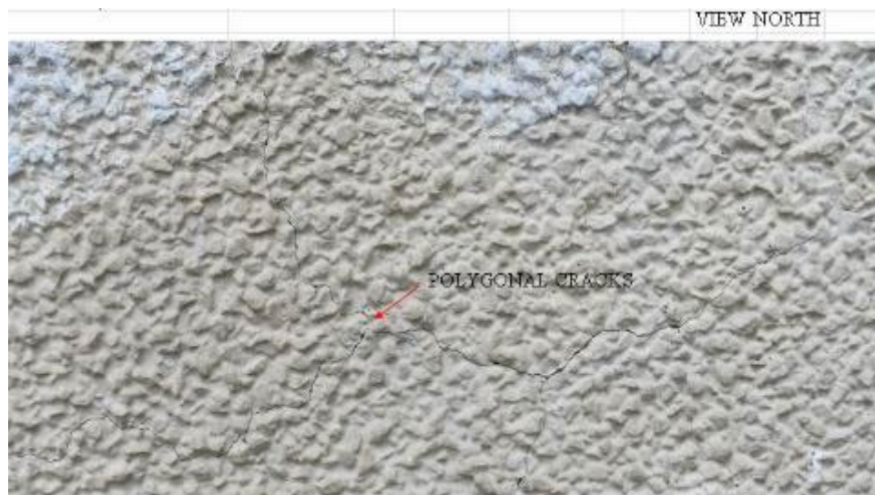
Figure 69. Polygonal Cracks (HL to 1/32 in) at STA 0+38, S. Wall, E. Abutment, Ledger Creek Bridge
