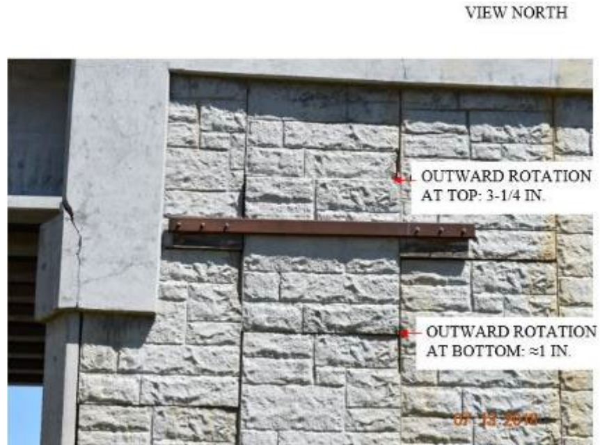
Figure 86. Close-up View of Displaced South MSE Wall, East Abutment of SH-33 Exit at US-20
