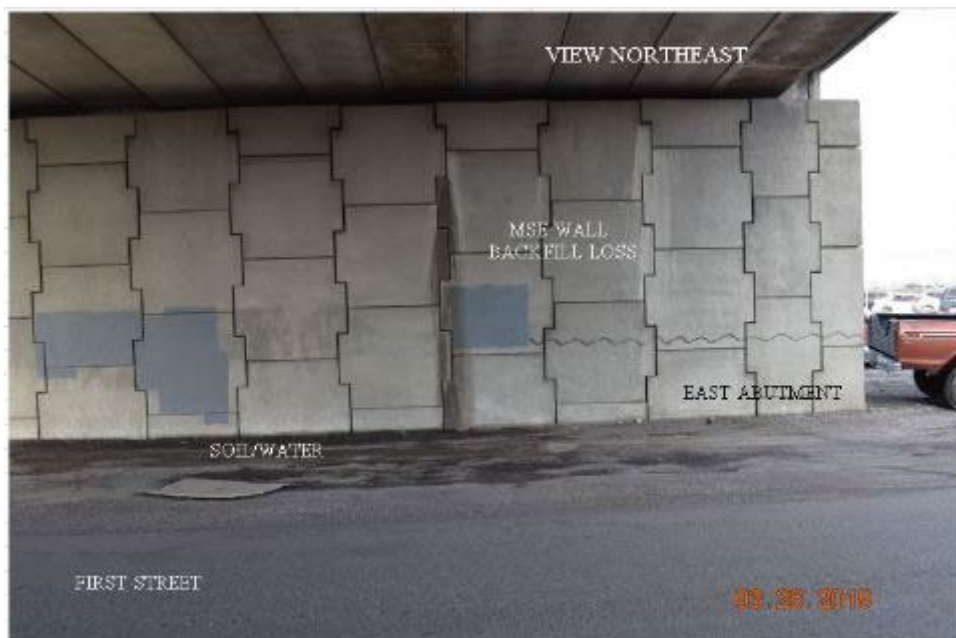
Figure 52. Backfill Loss, Gould Street Overpass, Wall 4
