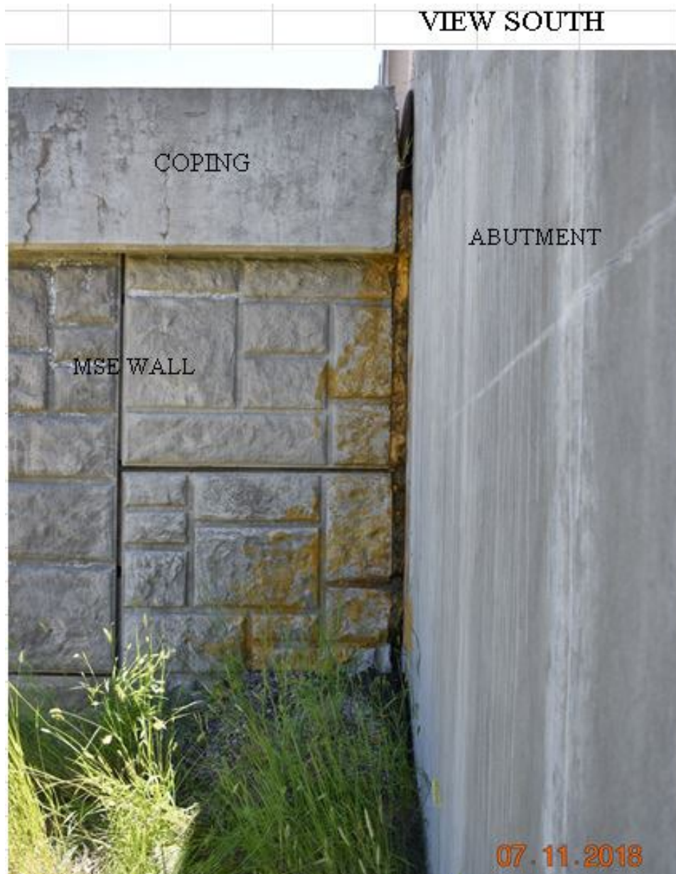
Figure 31. Photo of MSE Wall Damage at Interface with SE Abutment of Bitch Creek Bridge, SH-32
