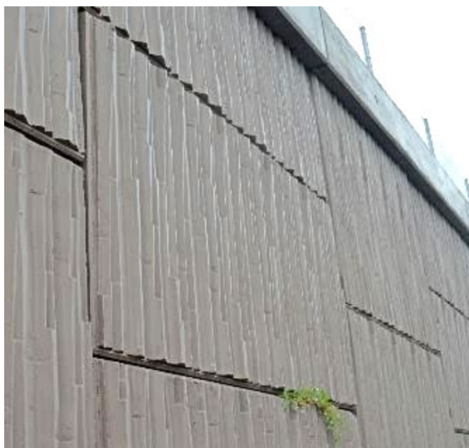
Figure 6. Rectangular Wall Panel with Bulge and Vegetation noted at L = 41 feet
