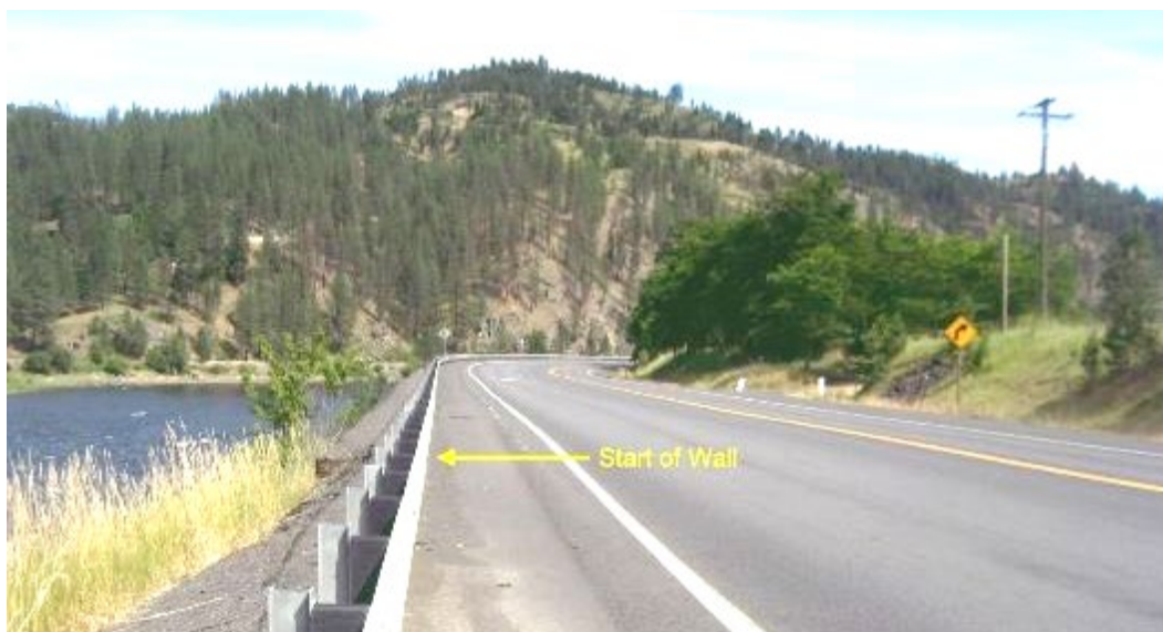
Figure 15. Western Wire Gabion MSE Wall at MP 53.00, WB US-12
