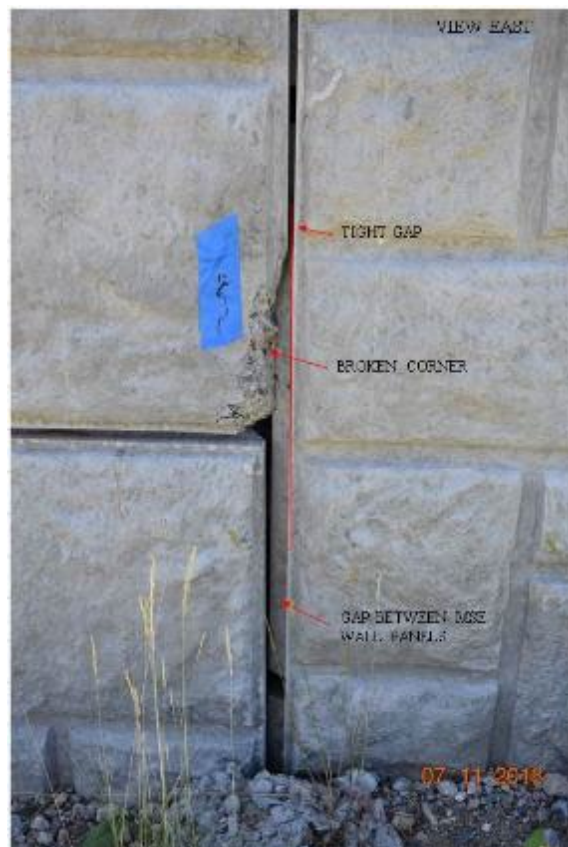
Figure 97. Broken Corner in East MSE Wall, South Abutment, at STA 0+17.1, Bitch Creek Bridge
