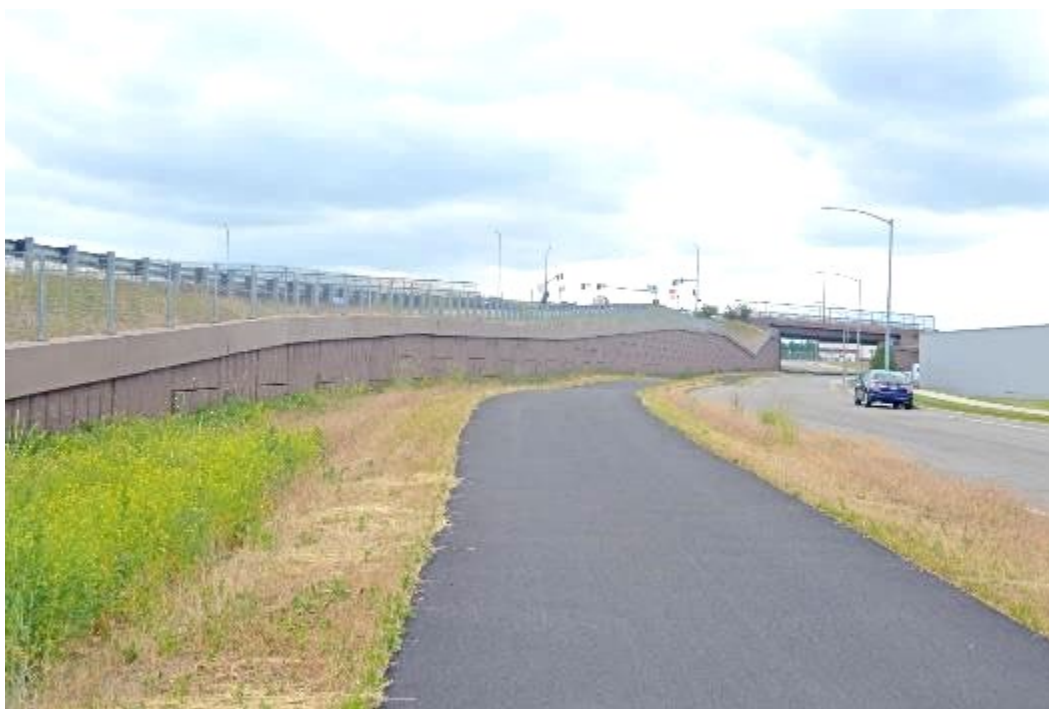
Figure 5. I-90 MSE Wall along the EB Off-ramp near MP 1.03
