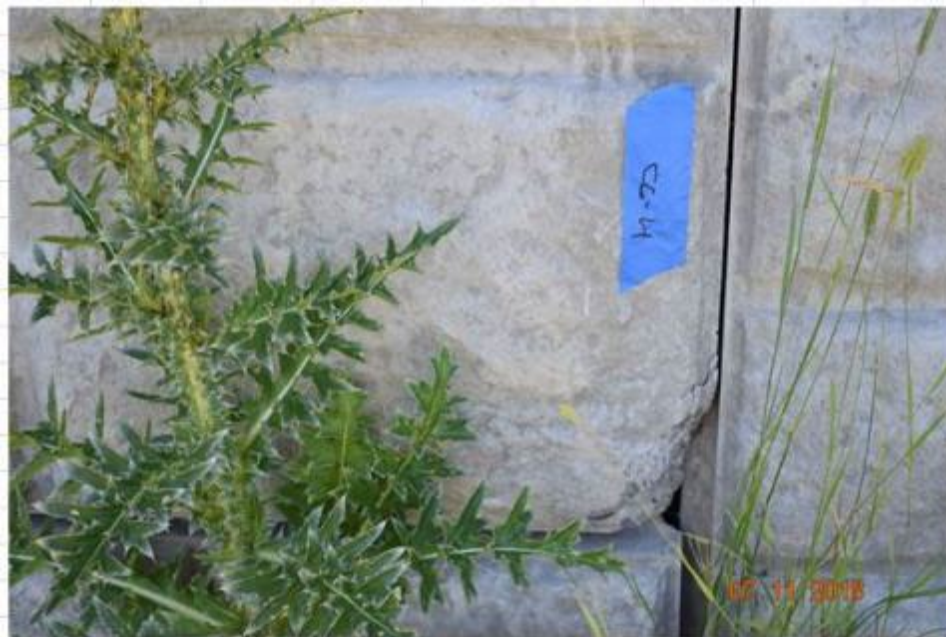
Figure 99. Broken Corner in E. MSE Wall, S. Abutment at STA 0+47.1, Bitch Creek Bridge
