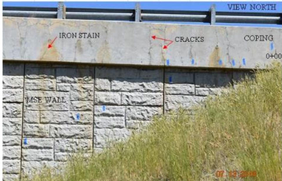
Figure 87. Close-up View of Coping Damage at S. MSE Wall, E. Abutment of SH-33 Exit at US-20
