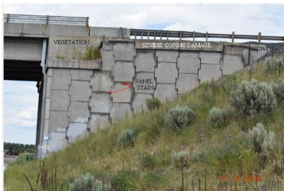
Figure 67. South Wall, East Abutment, Ledger Creek Bridge, Looking North
