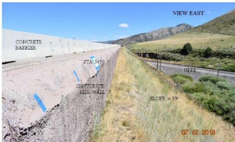
Figure 59. South MSE Wall, West Abutment, Topaz Bridge
