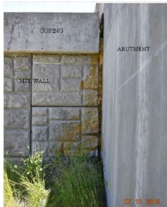
Figure 94. Lateral Displacement Damage at North End of South MSE Wall, Bitch Creek Bridge
