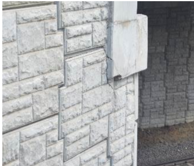
Figure 8. Typical “Cruciform” Concrete Panel and Damage in Bearing Wall at L = 110 ft
