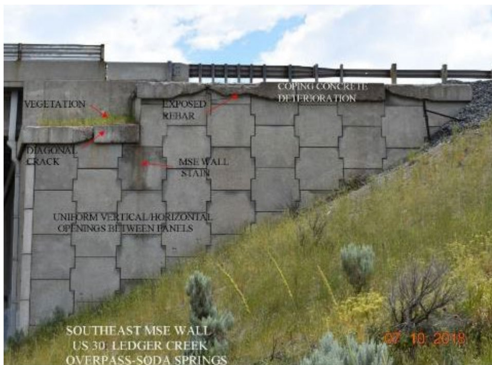
Figure 26. Severe Concrete Deterioration of MSE Wall Coping on Ledger Creek Bridge
