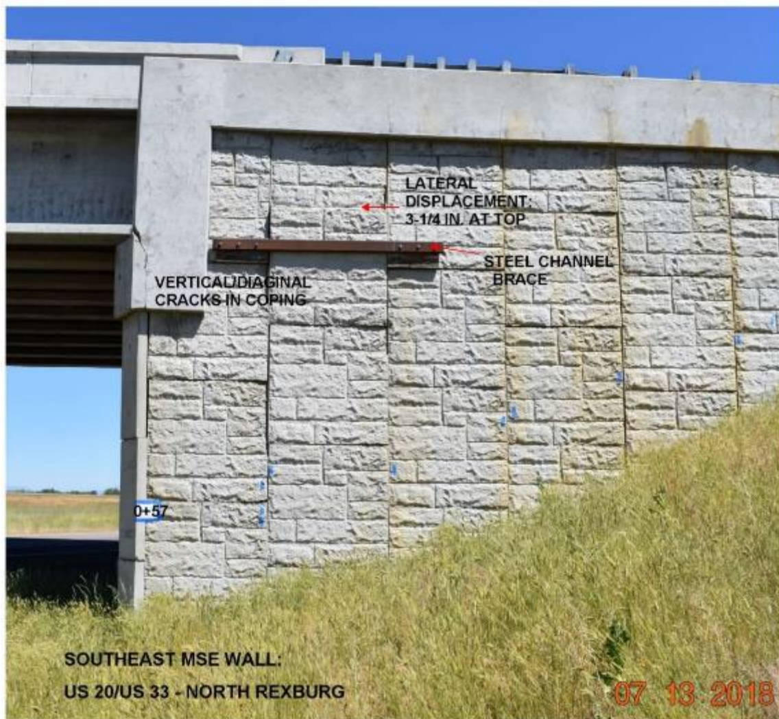
Figure 29. Lateral Displacement and Outward Rotation of MSE Wall Panels with Open and Tight Joints in Southeast MSE Wall at SH 33 Exit, US-20
