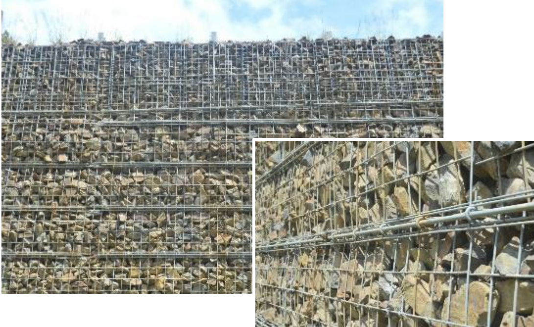
Figure 12. Wire-Gabion Configuration and Large Rockfill
