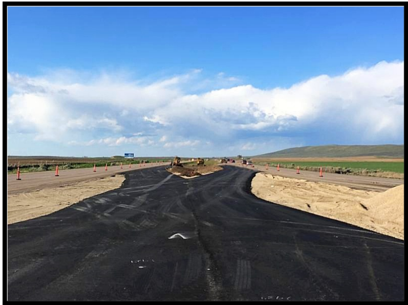
I-15 crossover near Fort Hall
